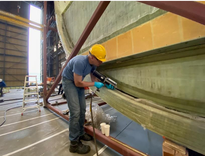
Sealing with Scigrip by BNS& ICC
