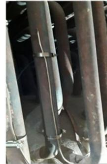
FBG sensors installation in some tubes of the superheated.
