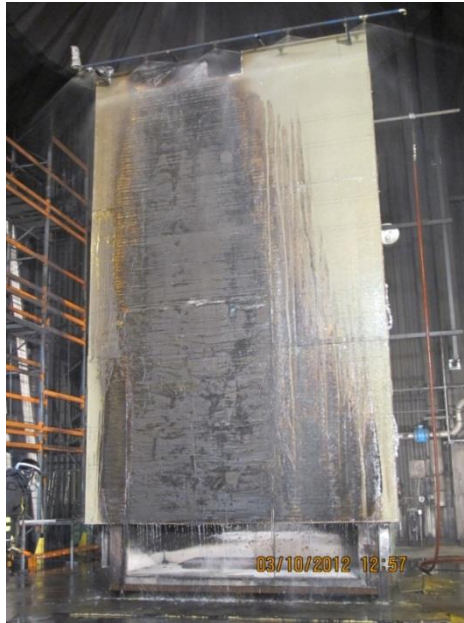
Figure 4.24. Fire damage on a FRP composite panel after a two minute fire exposure, representing a cabin fire through a balcony opening (structural integrity was lost throughout the whole height of the 6.5 m panel).
